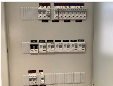
OK Electrical - sockets tested, operating
