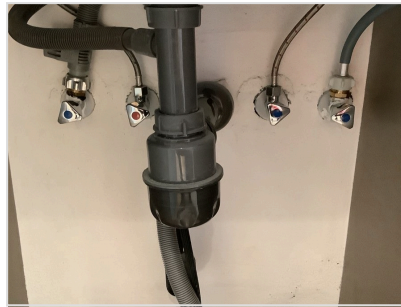
OK Under-sink drainage checked
