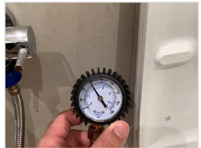
OK Water pressure checked
