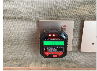
OK Living room sockets checked
